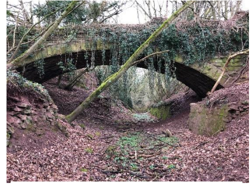
Bridge over the old GWR railway cutting.
