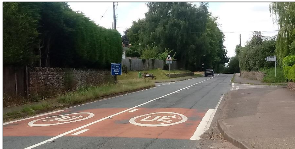
Existing road markings
